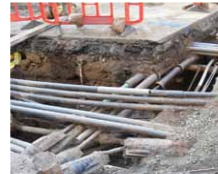
Figure 3. Typical congestion beneath our city streets
