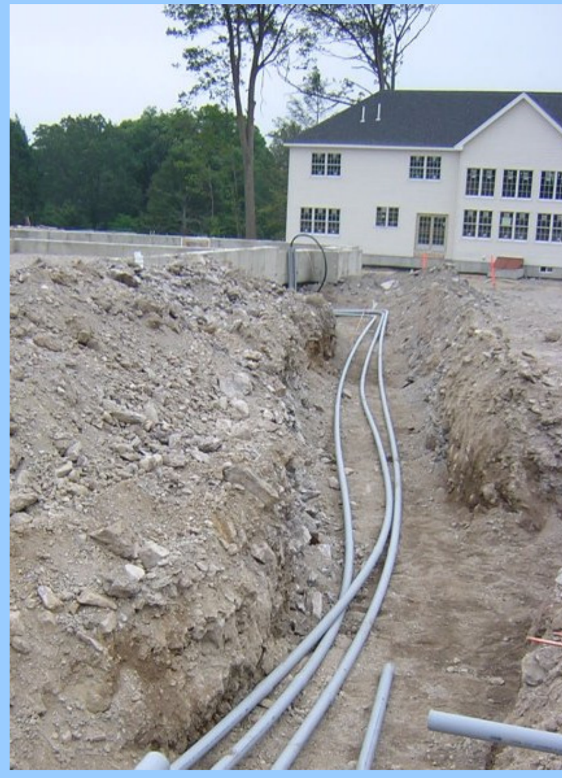
Figure 1: Laying the underground cable for a new road.
